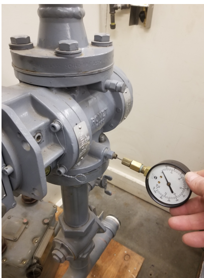
Figure 21 Two examples of pressure tests using P/T plugs. (Rod Lidstone) CC BY ( https://creativecommons.org/licenses/by/4.0/ )
